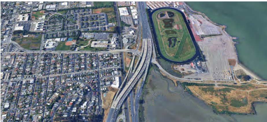
The I-80/I-580 freeways separate much of the city from its bayfront area. (Photo: Google Earth)
